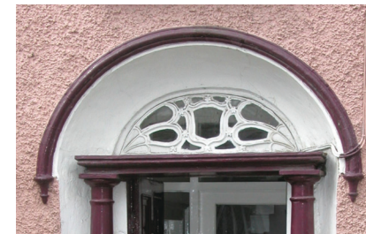
Barrack Street, NIAH 10400302
