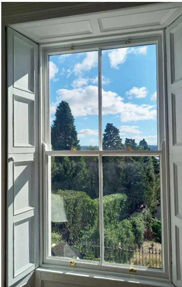
Figure 45: Two-over-two pane timber sash window
