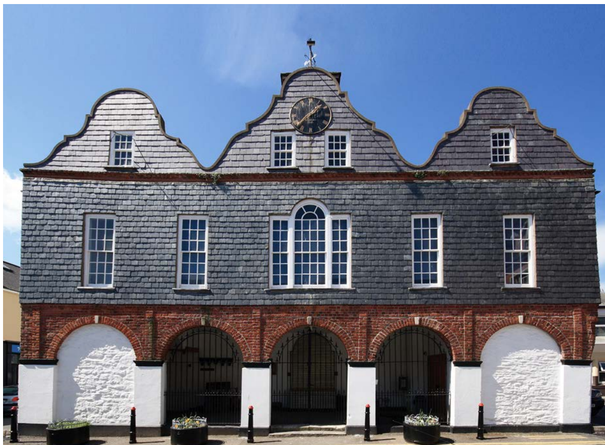
Figure 26: Natural slate hung front elevation
