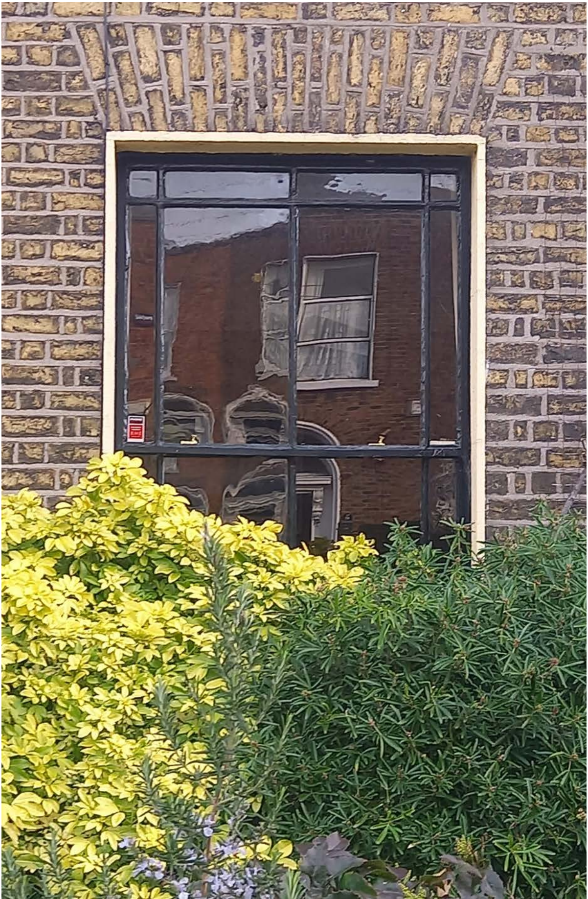
Figure 44: Timber sash window with original glass panes
