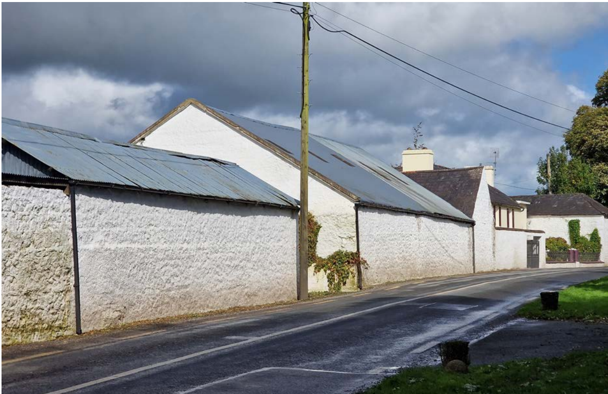
Figure 12: Limewash on traditional farm buildings
