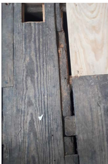
Figure 38: Care must be taken when lifting existing floorboards to conserve historic detailing like this biscuit joint
