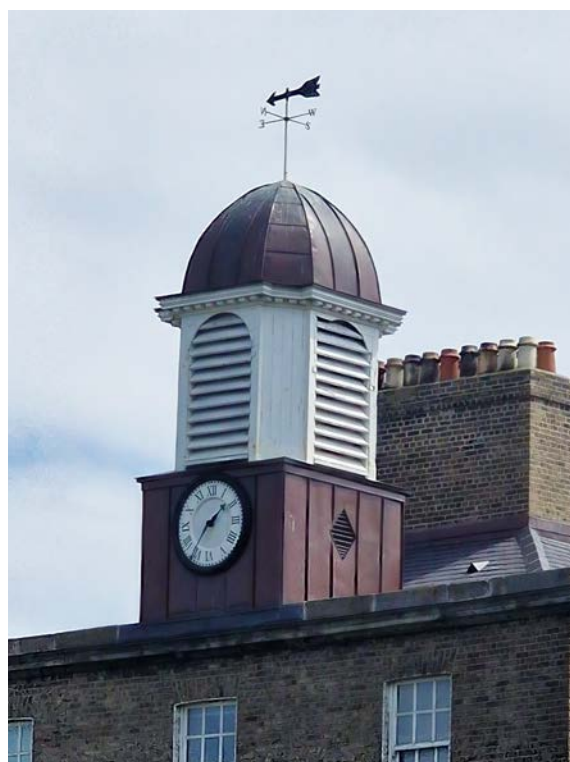
Figure 60: Copper-covered dome over louvred timber vent
