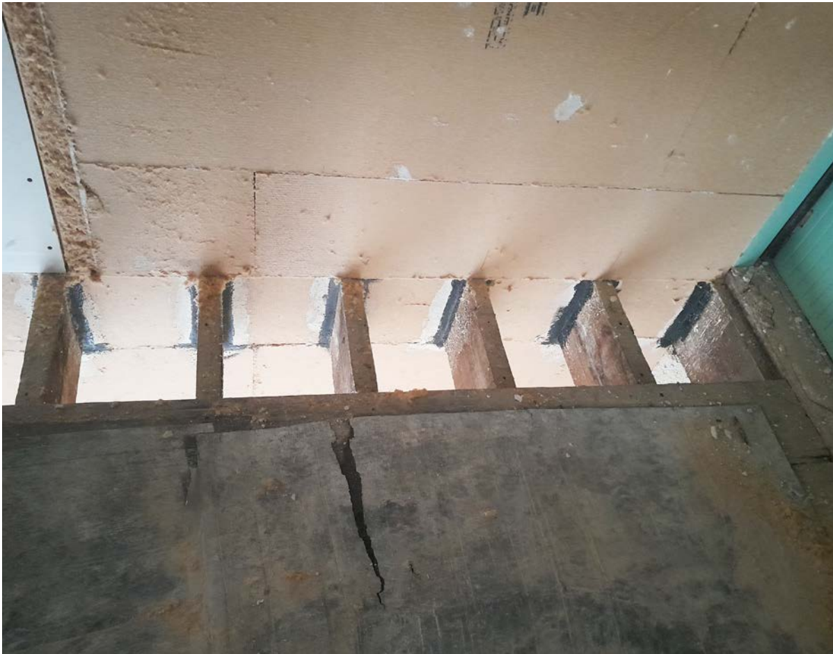
Figure 54: Woodfibre boards applied to walls and carefully fitted around and between floor joists to ensure continuity of insulation
