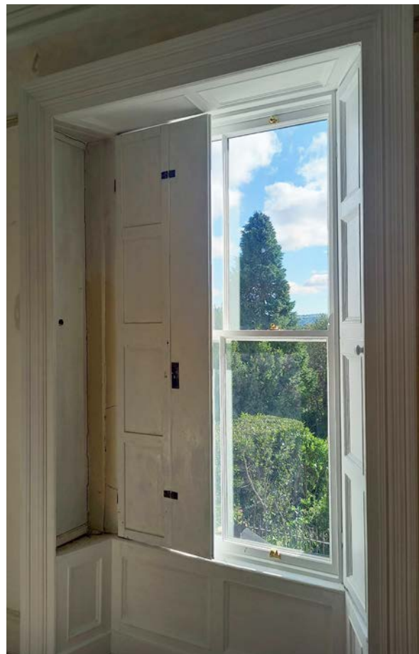
Figure 46: Two-over-two pane timber sash window showing operable shutters
