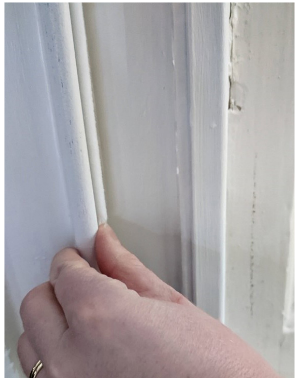
Figure 49: Discreet draught-proofing brush on a historic window
