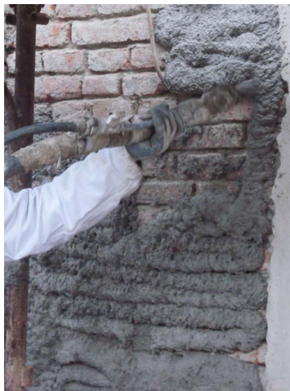
Figure 59: Insulating render spray applied on external walls. Spraying can use less material than application by trowel because the plaster is not being compacted.
