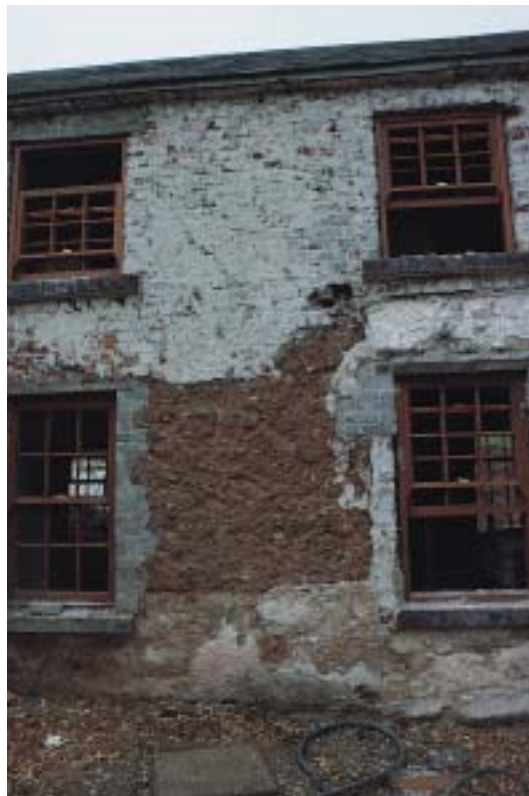
Exposed mud walling raised later in brick work.
