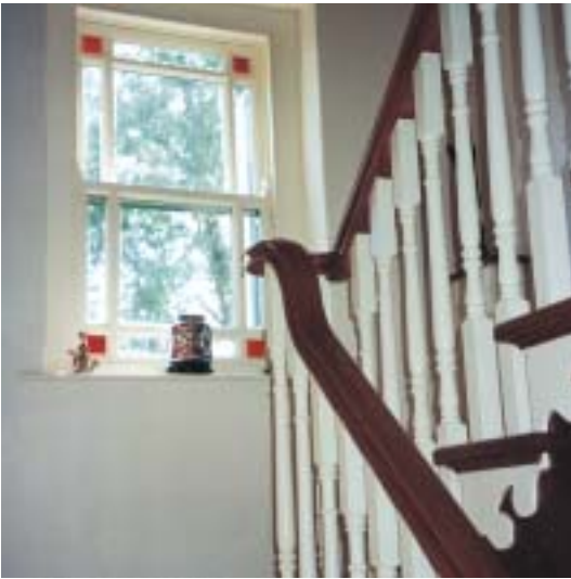
Open string stair.
