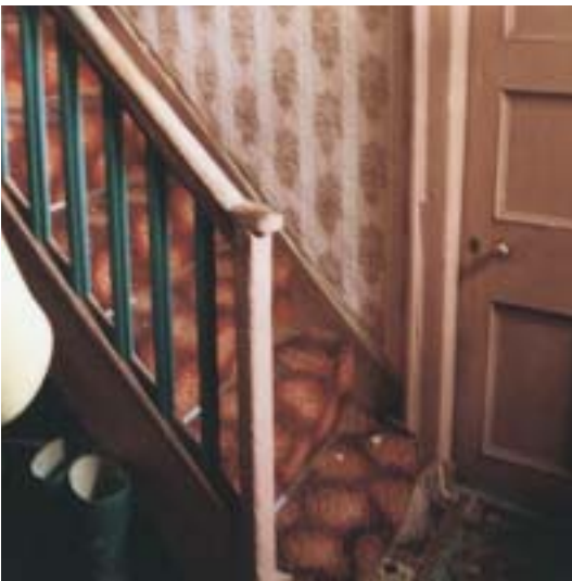
Closed string stair.
